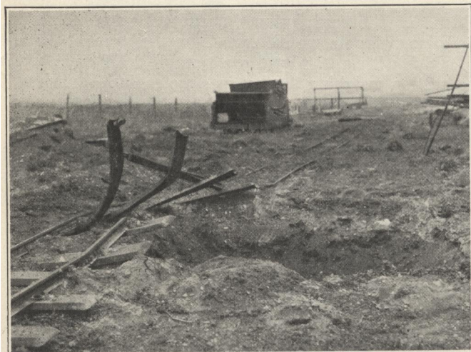
Signal Corps Photo. German 60-Centimeter Track Damaged by Bombs, Lancon, Ardennes, January 25, 1919
